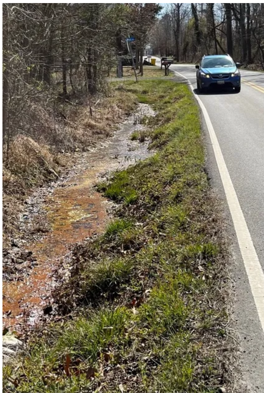
Source: Larry Brown | Route 261 in Holland Point doesn't have a shoulder
